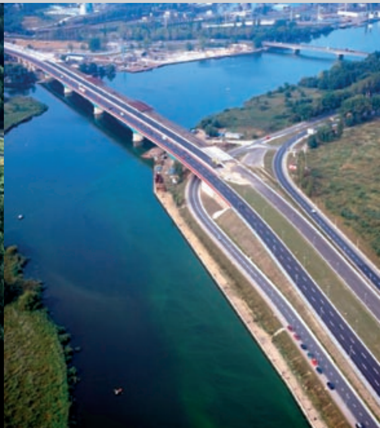
Bridge across the Regalica River
