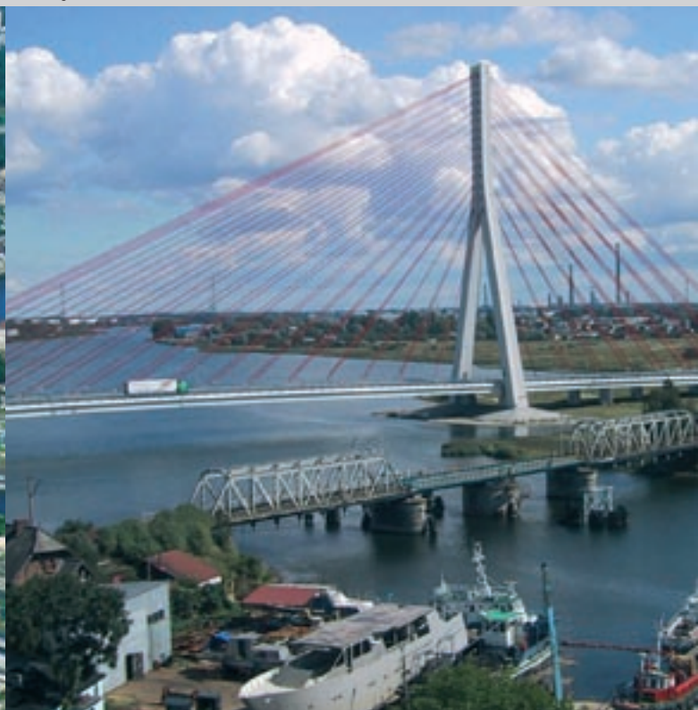
New Bridge in Gdansk
