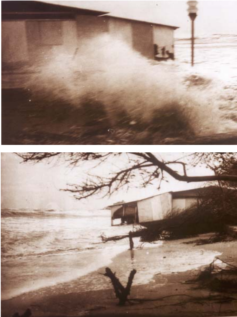
Fig. 9: Storm damages on Mamaia beach 1986.
