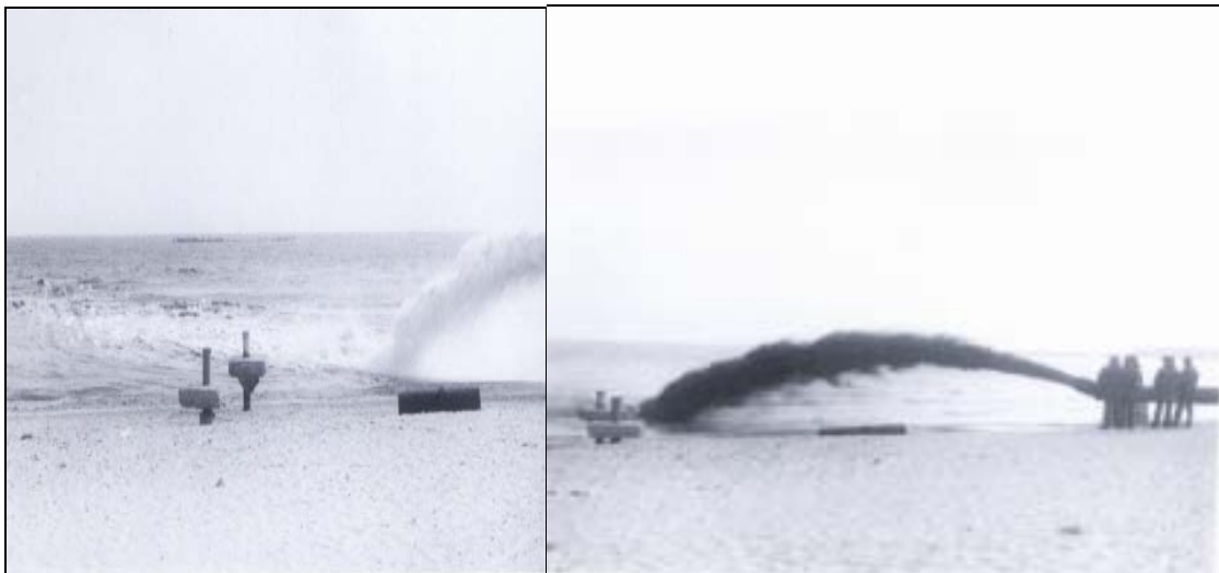
Fig. 11: Pumping sand from Siutghiol Lake - artificial nourishment.
